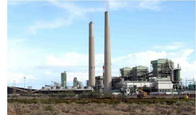
CHOLLA POWER PLANT
